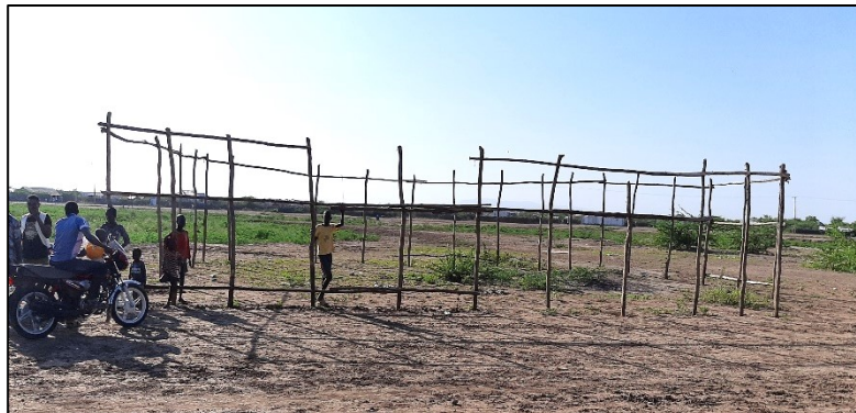
Beginnings of church building by Refugee Camp Church of Christ
