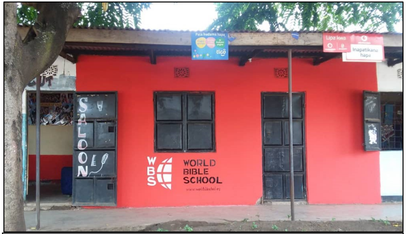
The newly painted WBS Service Center in Monduli, Tanzania
